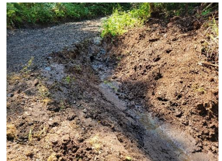
Culvert Installed on Cougar
